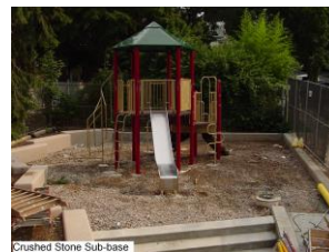
Crushed Stone Sub-base
