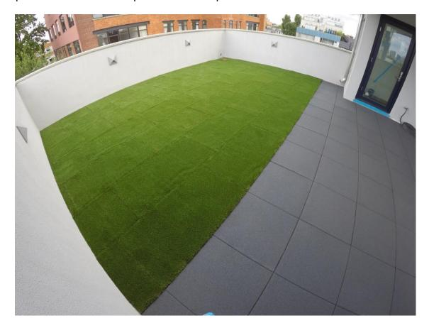
This particular roofing project incorporated the use of our NEW 1 3/4" thick Turf-Top tile in conjunction with our standard 2" thick rubber paver known as our Pave-Land series in order to have a seamless transition for one type of surfacing material to the next.
