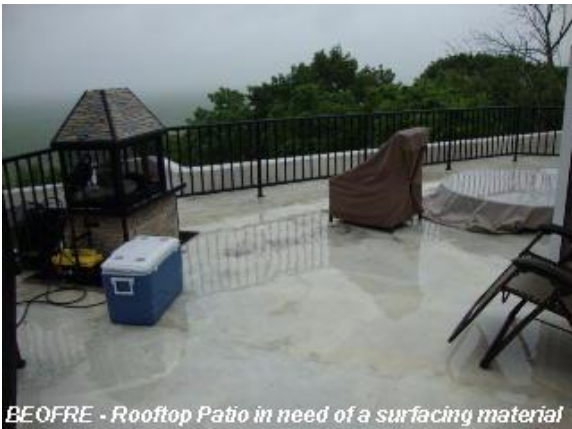
BEFORE - Rooftop Patio in need of a surfacing material
