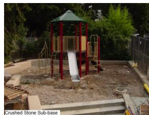
Crushed Stone Sub-base
