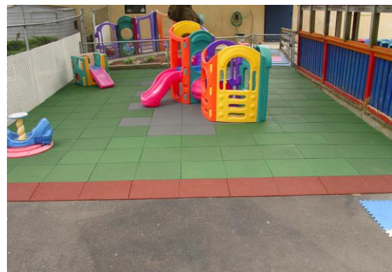
AFTER - 500 sq. ft. play area w/new safety surfacing & ADA ramps
